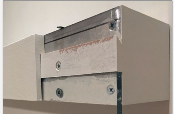
Optium® sheet hangs from the top bracket by securing machine screws through the acrylic into the aluminum. Photo courtesy of the Cantor Arts Center at Stanford University.
