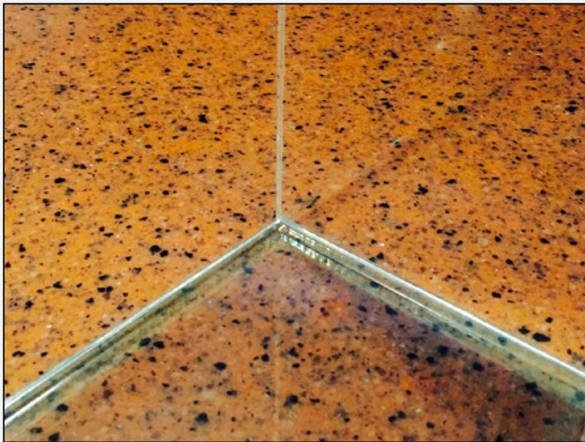
Close-up of the inside of the glass bonded corner. © JIT Companies Inc.
