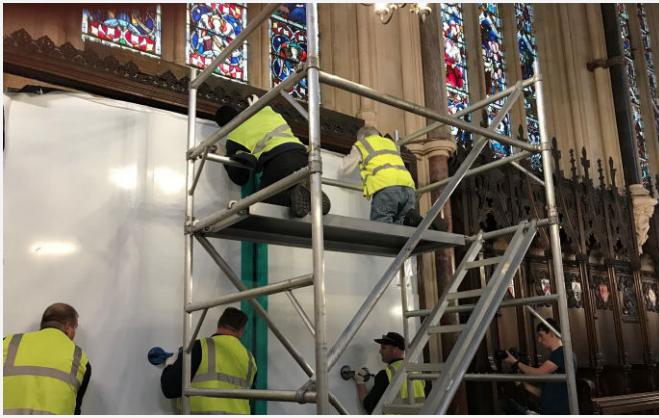
Installation of Optium Museum Acrylic® into the wall frame.
